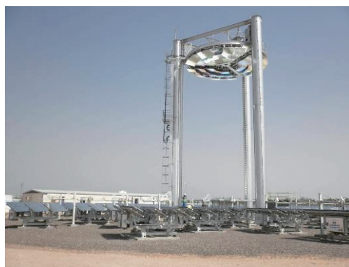
Photo 1 100 kW beam-down CSP installation in Abu Dhabi.
